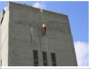
**The outcome:** Both structures within the RAF Leeming station were remediated against all areas of cracked and spalling concrete, with any leaking cracks chased out and filled, before completing the roof repairs. The application of a guaranteed reinforced waterproof
